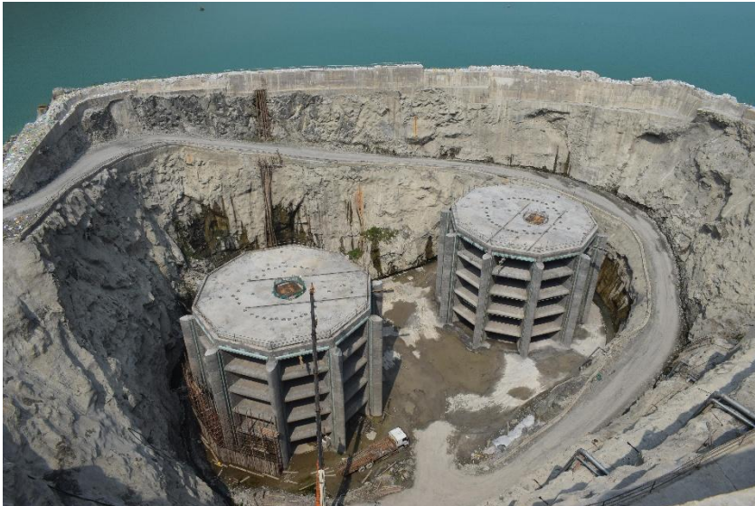
Raised intake structures for the Tarbela Dam 4th Tunnel (left) and 3rd Tunnel (right) behind a cofferdam formed from natural rock (below) and concrete (above and in the process of demolition), prior to screen fitting.
