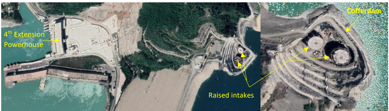
Raised intake structures under construction for the Tarbela Dam 3 rd and 4 th Tunnel behind a cofferdam formed from natural rock (below) and concrete (above).
